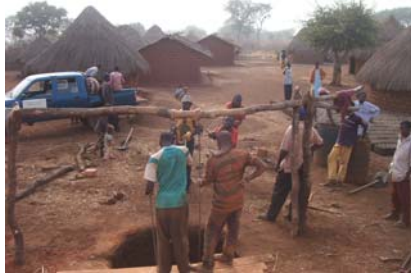
The work site during well installation
