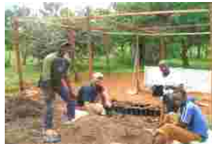
Nursery construction begins
