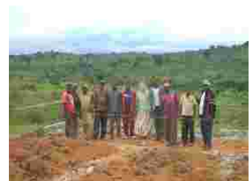
The construction team completes the house footer
